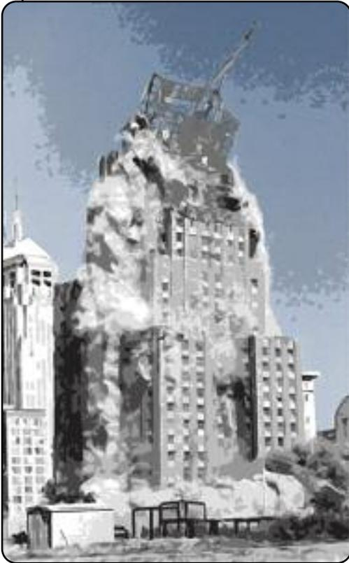
*Controlled demolition of abandoned buildings creates tons of rubble. If graded and sized properly, this waste material can be used as a substitute for native gravel in drainfields.*
