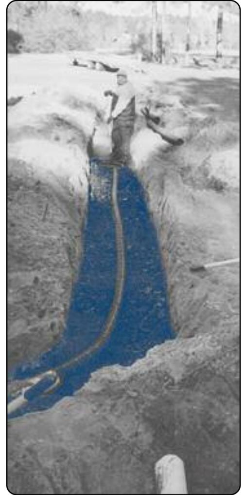
*Bottom layer of trench with six inches of tire chips and four-inch pipe.*
