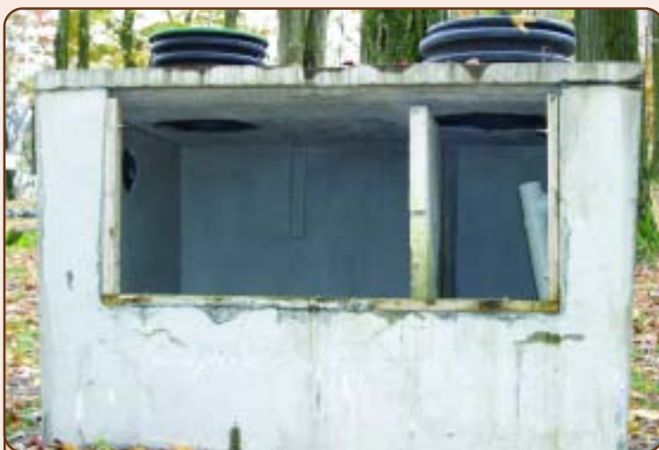
Figure 3 Two-compartment septic tank with risers. Note: The hole is for viewing purposes.
